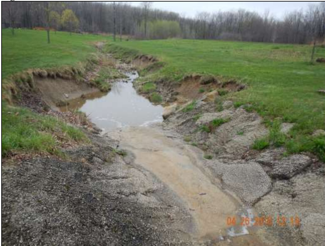
Figure 23. Stream restoration: Before
