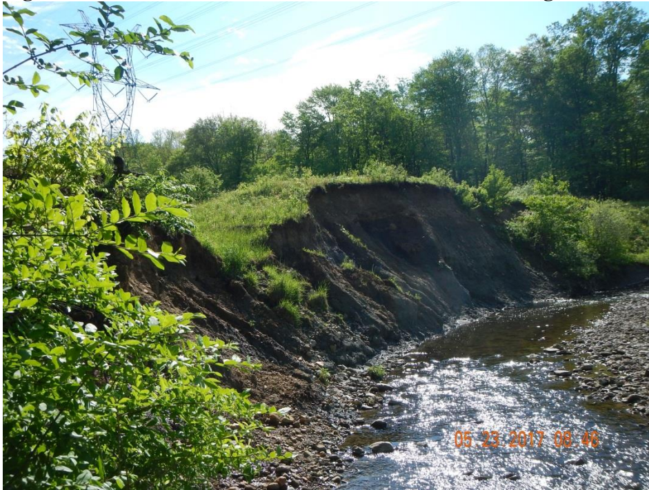
Figure 37. Streambank Erosion and Sedimentation on Big Creek
