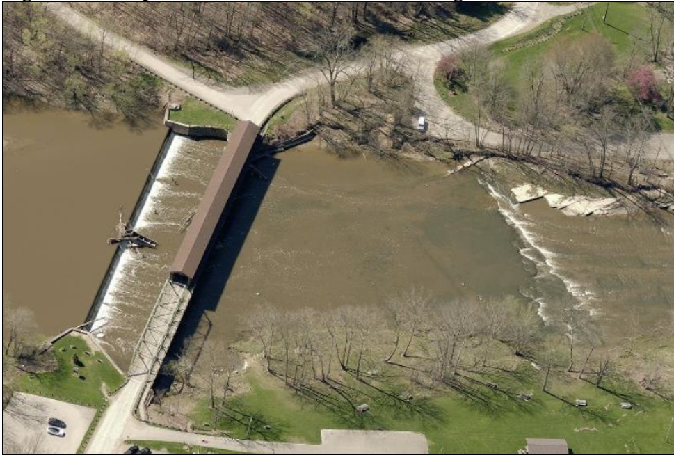
Figure 19. Harpersfield Dam and Covered Bridge
